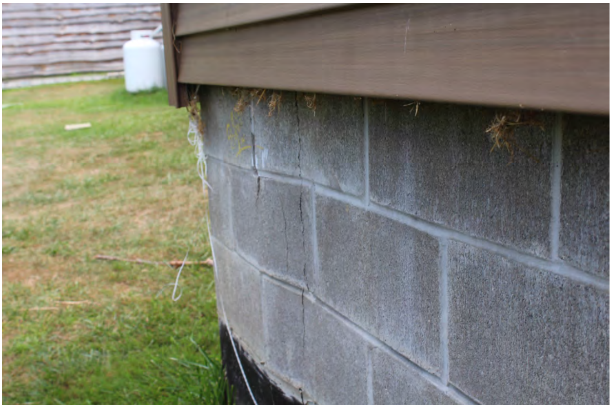
3028, 8/15/2022, by Sam Gowan: View of the caved in basement wall at the northeast corner of the southwest wall of the addition at 445 Scribner Road.
