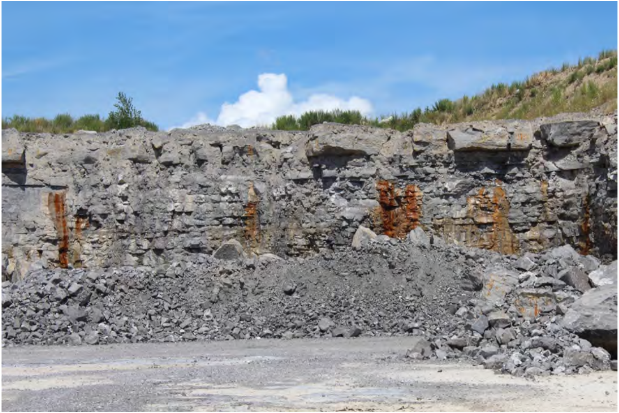
3062, 8/15/2022, by Sam Gowan: Ground water seepage on the north highwall, northeast corner of the County Line Stone Akron Quarry.
