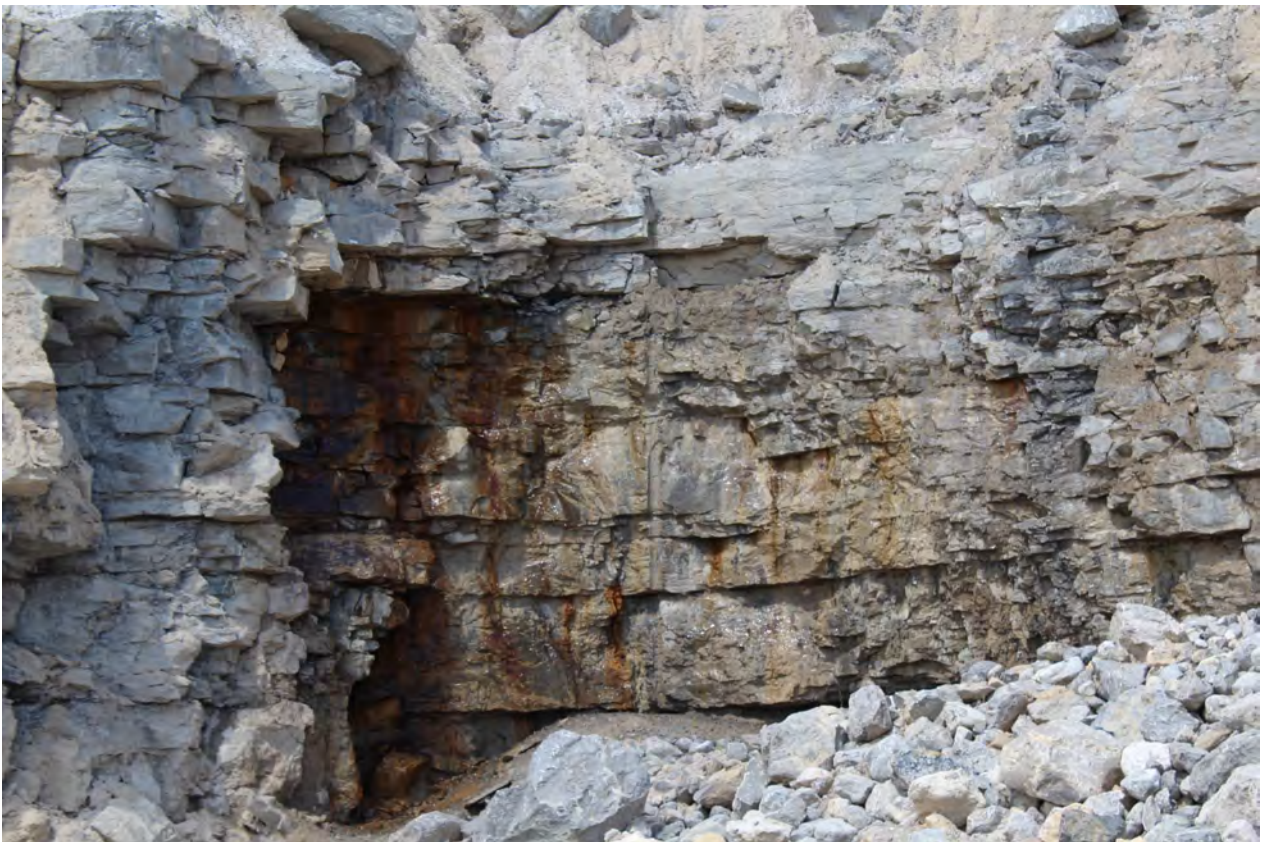
3057, 8/15/2022, by Sam Gowan: Ground water seepage from a few feet below the base of the overburden in the north face of the highwall at the County Line Stone Akron Quarry.
