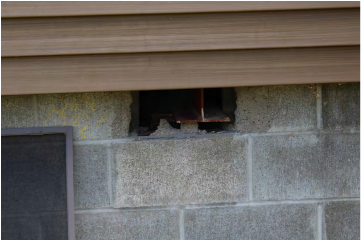
3033, 8/15/2022, by Sam Gowan: Steel beam visible pushing through the northwest wall of the addition at 445 Scribner Road. View to the east.
