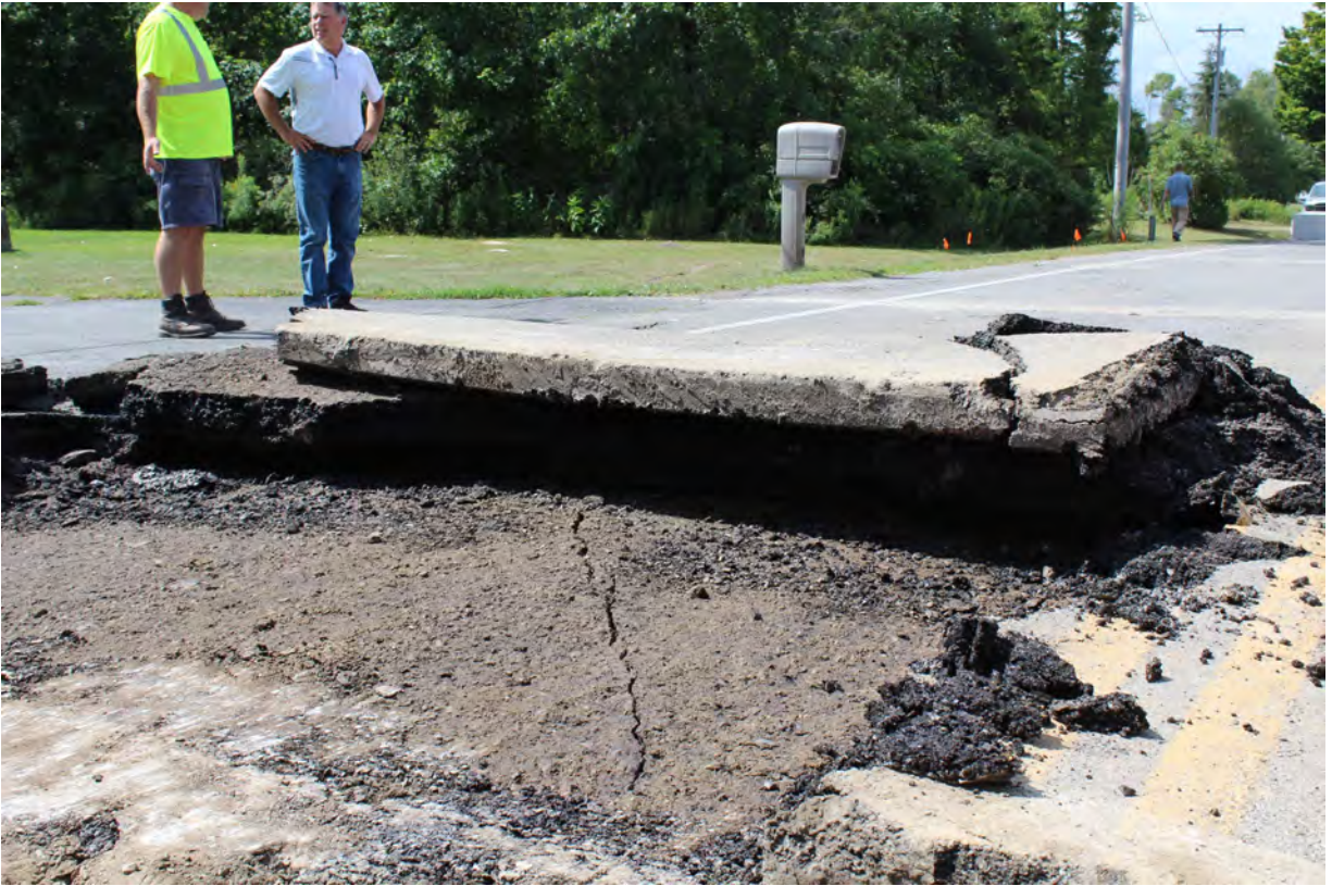
3017, 8/15/2022, by Sam Gowan: View to south-southwest of a fracture in the subbase of Scribner Road with Norm Gardner (white shirt) of CPL and the mailbox at 440 Scribner Road in the background.
