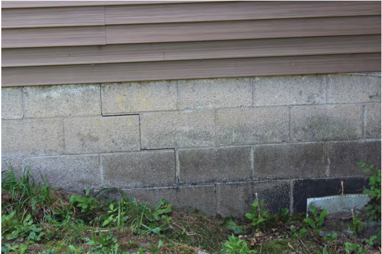
3031, 8/15/2022, by Sam Gowan: View to the east of the northwest foundation wall of 445 Scribner Road. Fracture is in the northwest basement wall to the northeast of the addition.
