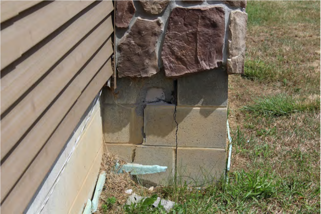
3038, 8/15/2022, by Sam Gowan: View to the northeast of broken and fractured cinder blocks on the southeast side of the addition at 445 Scribner Road.
