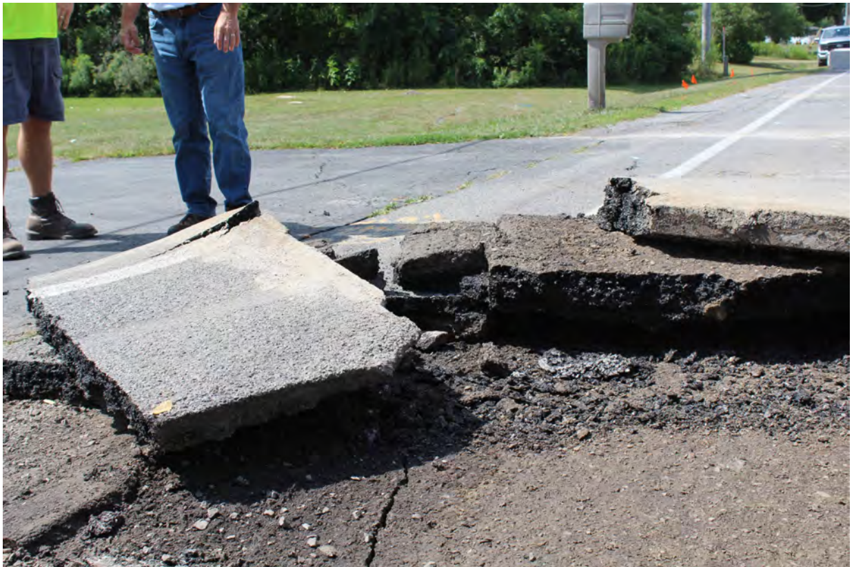
3018, 8/15/2022, by Sam Gowan: View to the south-southwest of a fracture in the road subbase.
