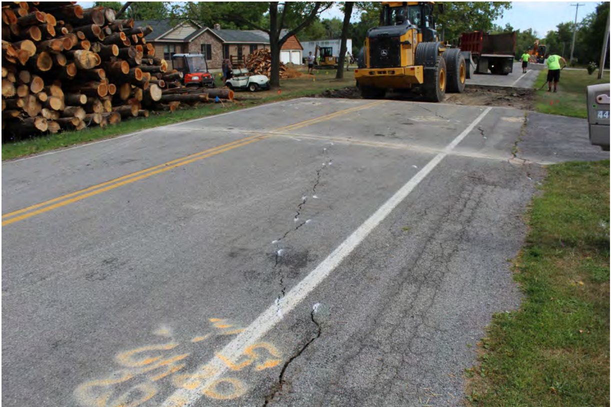
3009, 8/15/2022, by Sam Gowan: View to the north-northeast. 445 Scribner Road (Corfu, NY) on left side of road. Large woodpile recently placed at 445 Scribner Road. Fractures from recent event extending diagonally across the road.
