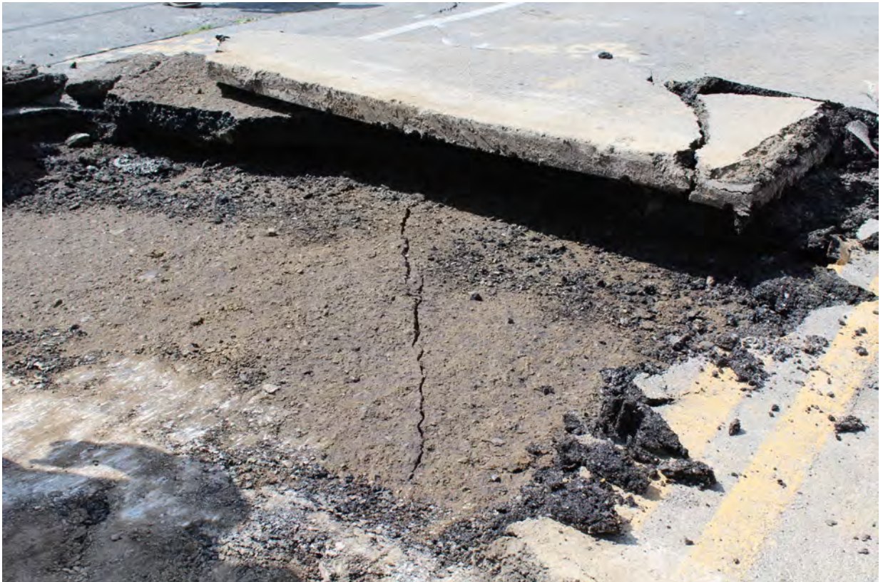
3016, 8/15/2022, by Sam Gowan: View to the south-southwest of a fracture in the recently exhumed subbase of Scribner Road
