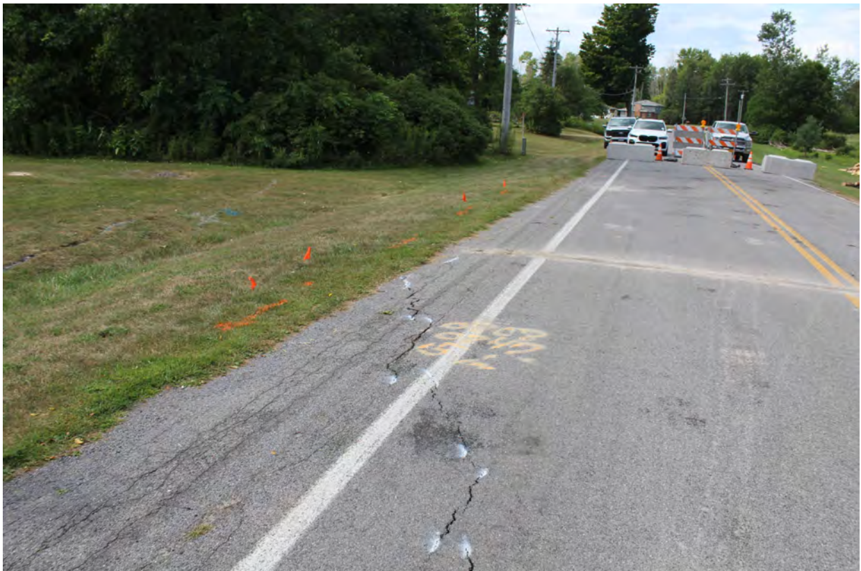
3010, 8/15/2022, by Sam Gowan: View to south-southwest across the corner of the yard at 440 Scribner Road. Fractures visible on both sides of the roadside ditch.
