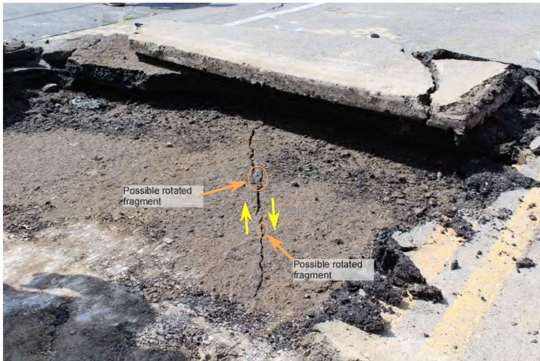
FIGURE 16 Scribner Road Fracture in Road Base Below Pavement Scribner Road Project County Line Stone Town of Pembroke Genesee County, New York
