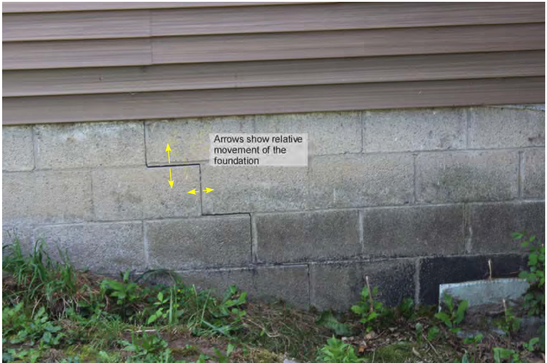
FIGURE 19 Fracture and Relative Movement of Basement Wall at 445 Scribner Road
